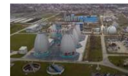
Figura 8 – Vedere SEAU Glina 2023 ( https://ziare.com/statie-epurare-glina/finalizare-proiect-statie-epurare-glina )
